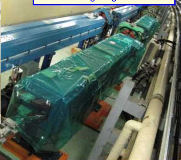
Installation of 100 new long LER bending magnets
