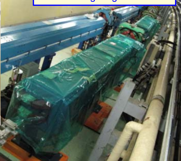
Installation of 100 new long LER bending magnets
