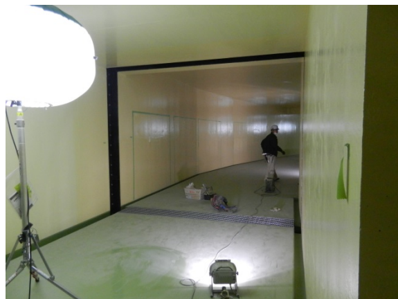
Inside DR tunnel
