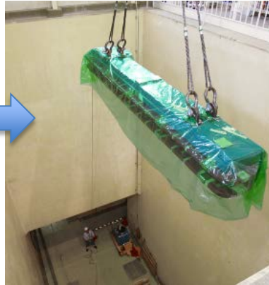
move into tunnel
