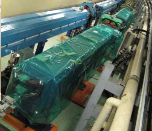
Installation of 100 new long LER bending magnets
